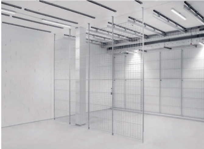
Fixed freestanding mesh panels
